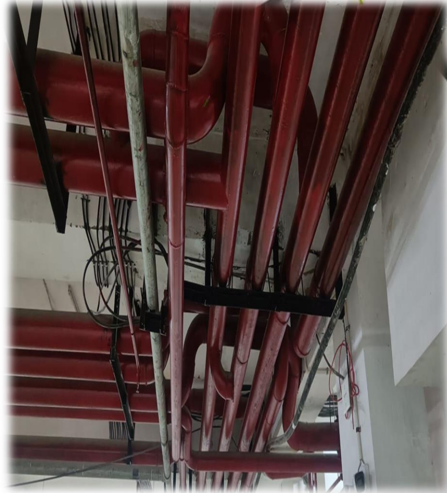
Basement Work Northern Railway Chanakyapuri Site New Delhi (India)
